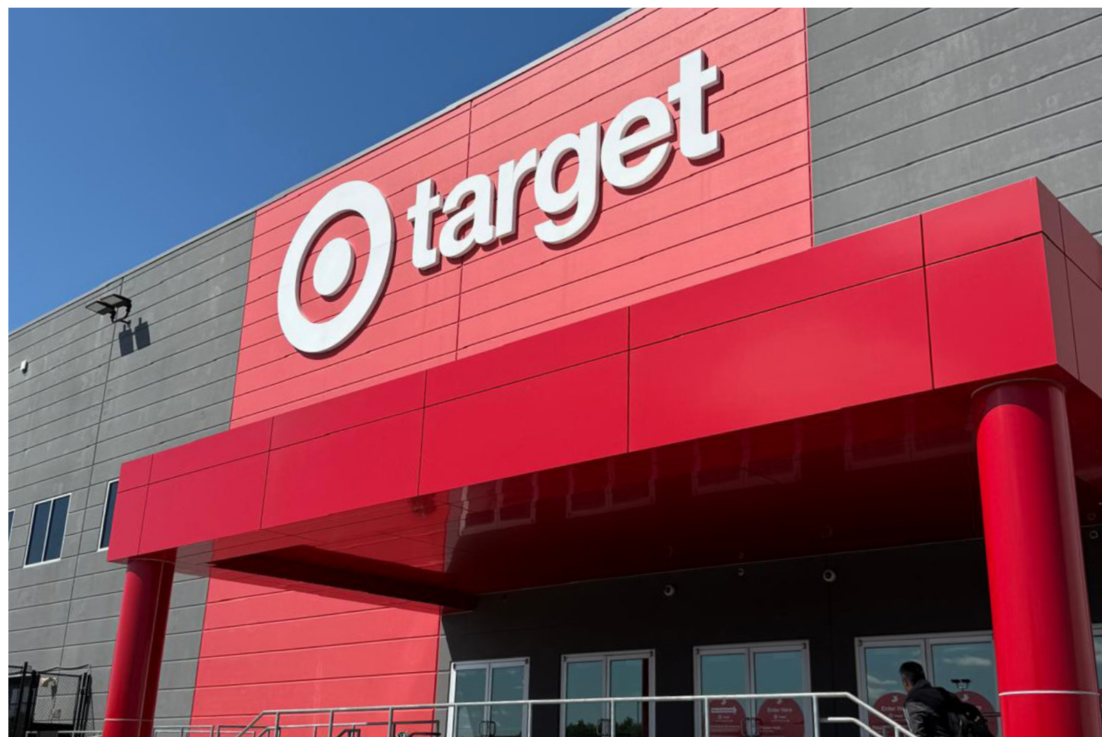
Entrance to Target Flow Center in Logan Township, NJ
