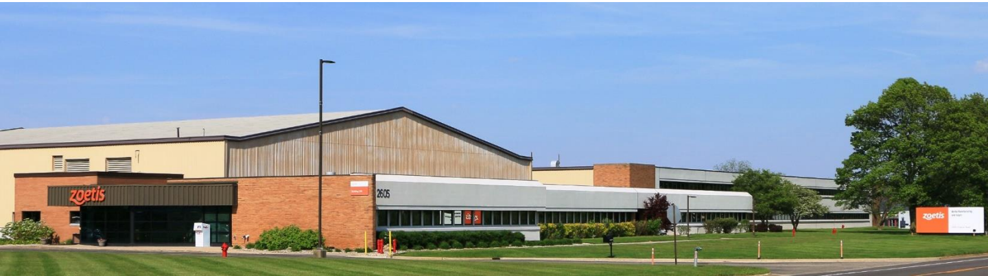
View of Zoetis' Kalamazoo GMS facility
