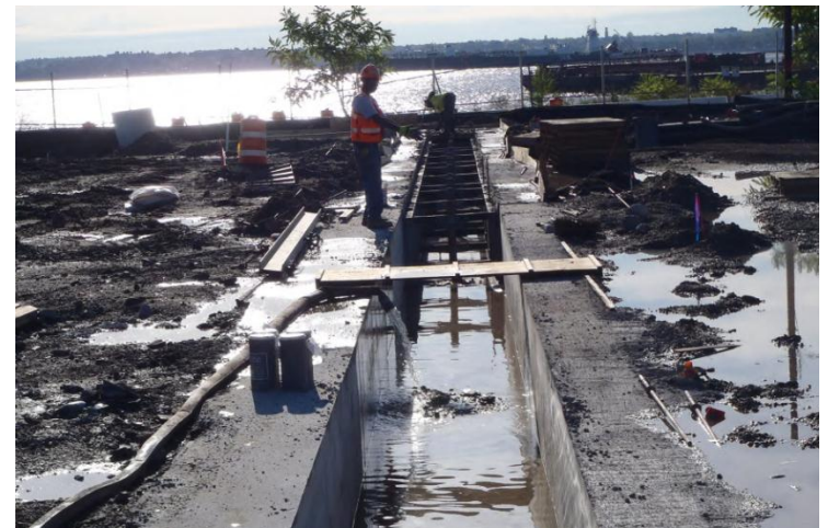
Water Siphon under construction
