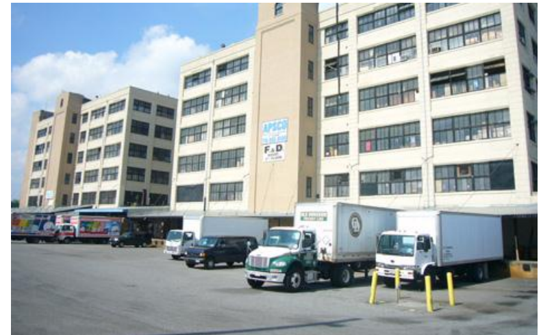
Bush Terminal Industrial Campus
