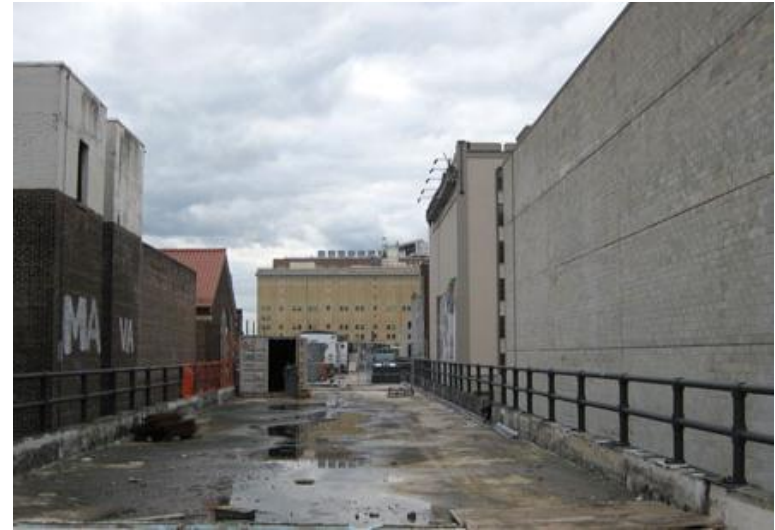
High Line before construction
