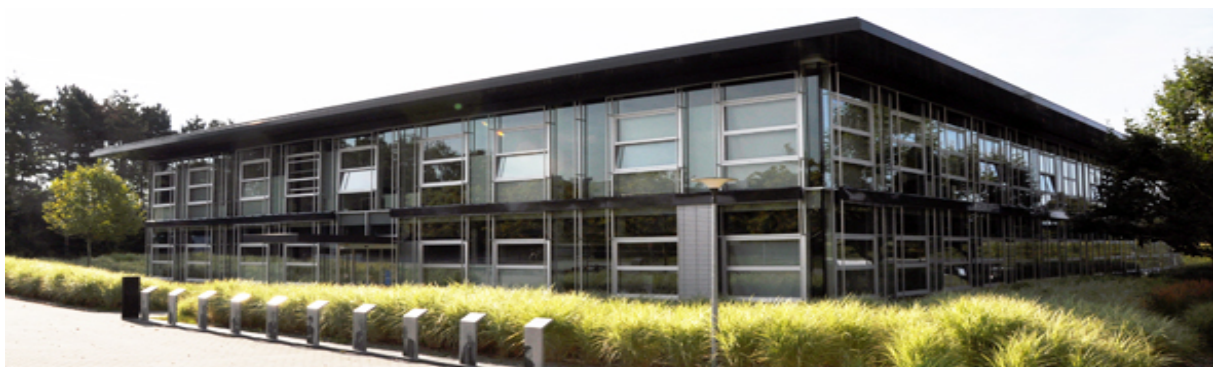
Extranef building in the Quartier Chamberonne of the University of Lausanne
